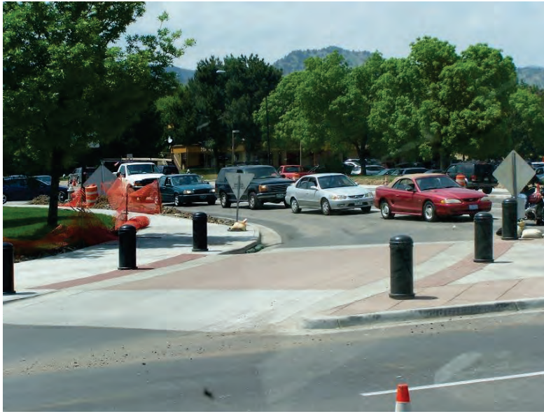
Figure 77 | Raised Crosswalk at Channelized Right Turn
