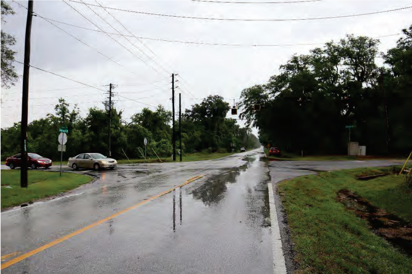
Looking north into the intersection along Culbreath Road
