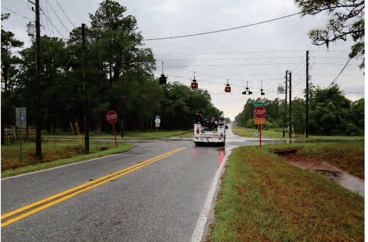
Looking west into the intersection along Hayman Road
