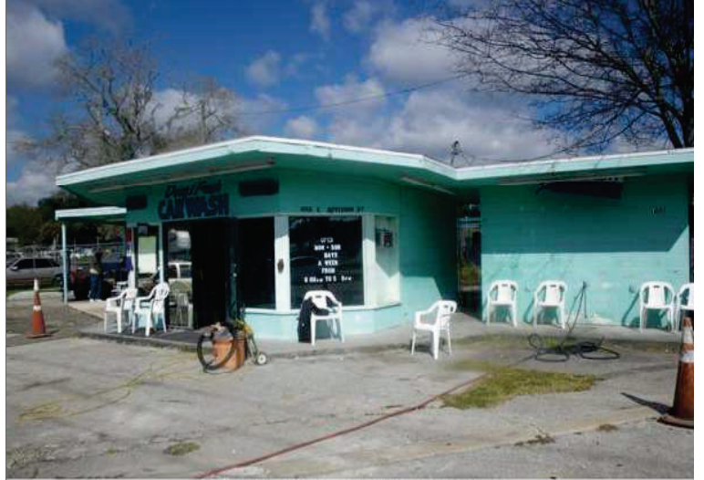
February 2015 BUILDING 01 PHOTO
