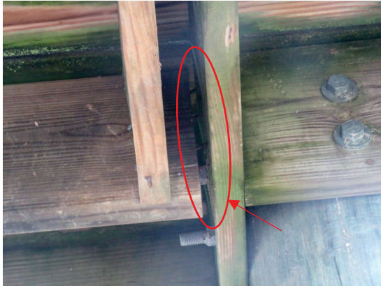
Exhibit 9 – Separation of end-nailed joist connection
