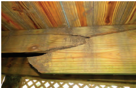
Exhibit 2 – section loss/separation along deck joist
