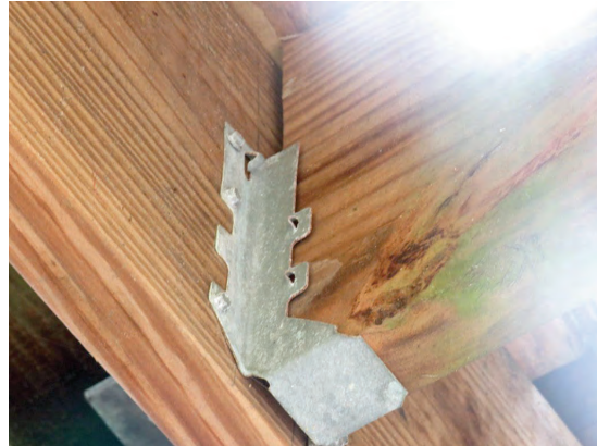
Exhibit 10 – Metal joist hanger
