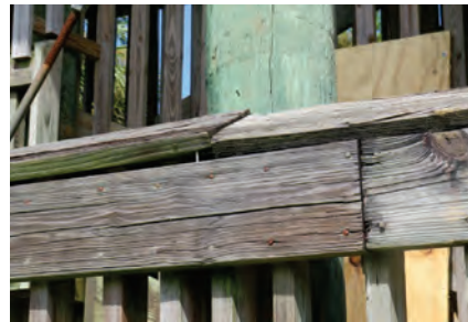
Exhibit 3 – deteriorated railing components
