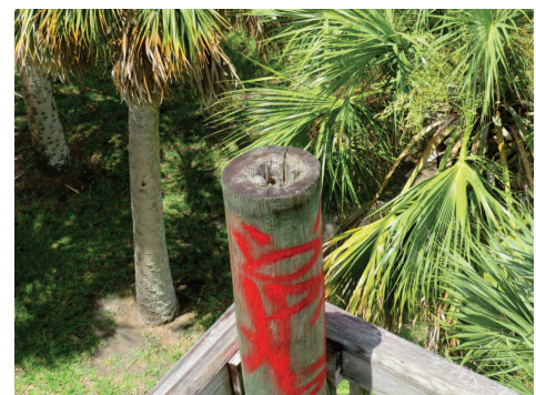
Exhibit 6 – Pole top deterioration
