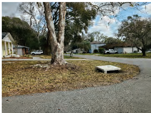
Figure 3: Drainage Inlet at Dakota Drive/Wakefield Drive NE Quadrant
