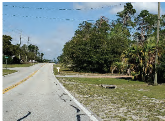
Figure 4: Drainage Inlet at Freeport Drive/Elkin Ave SE Quadrant
