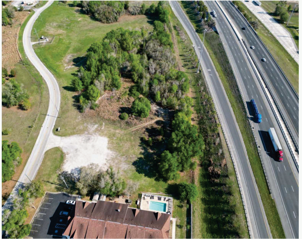
Eastern parcel frontage along Nature Coast Blvd
