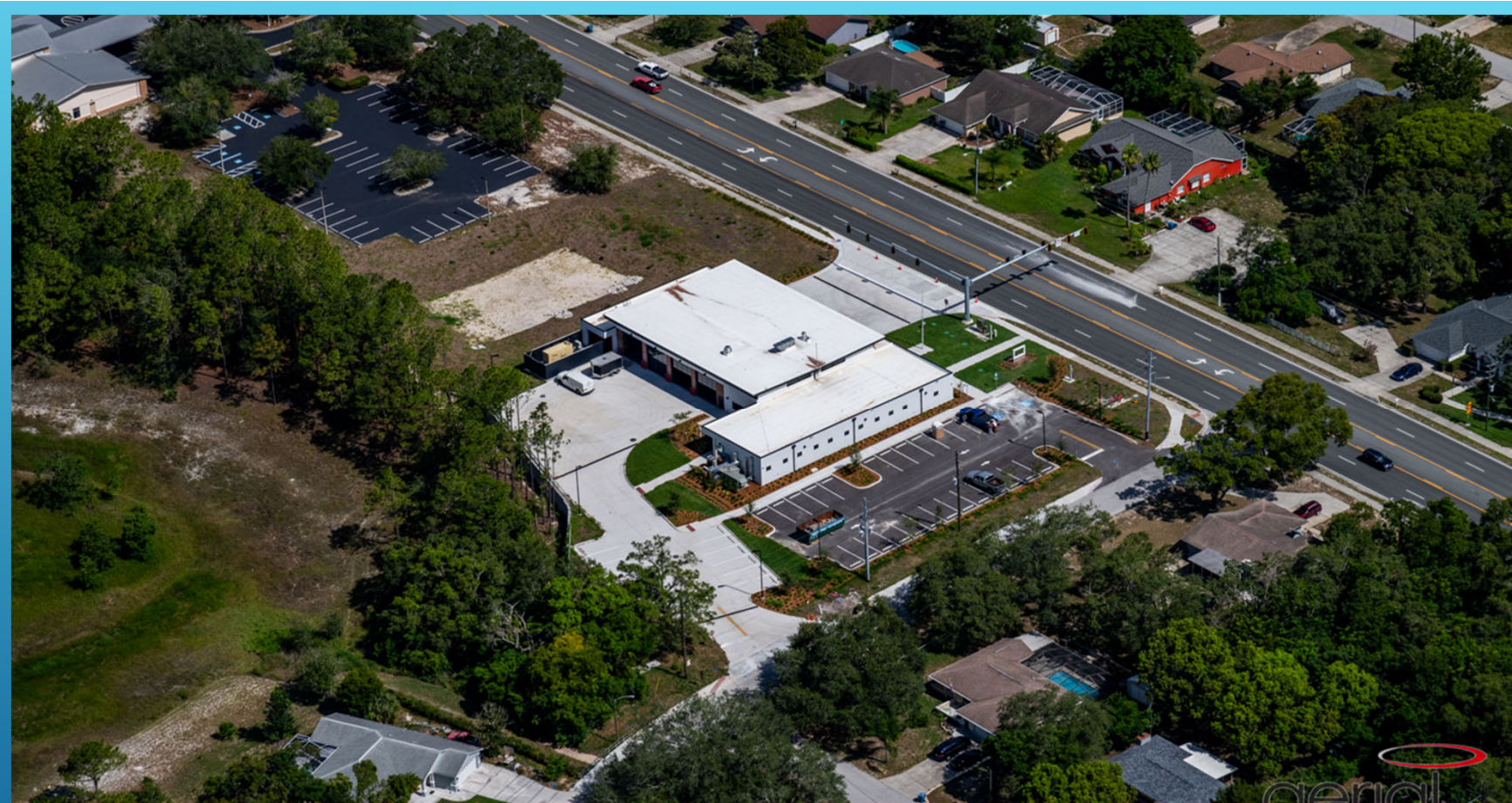
FIRE STATION 5 SPRING HILL DRIVE
