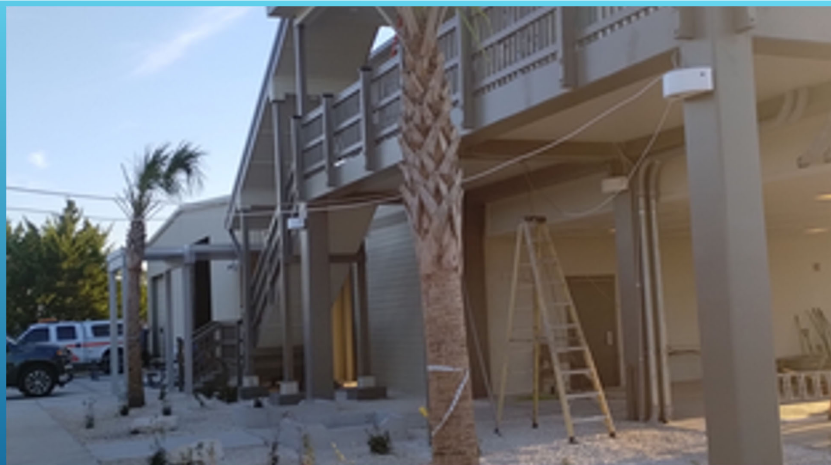
FIRE STATION 6 HERNANDO BEACH
