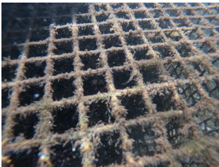
Figure 1. Example of biofouling prior to removal.
