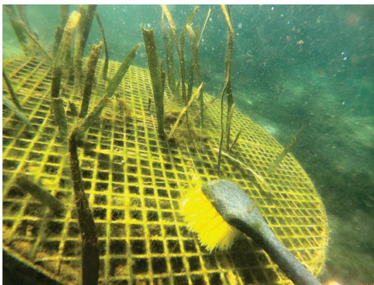
Figure 2. Example of Sea & Shoreline biologist removing biofouling.
