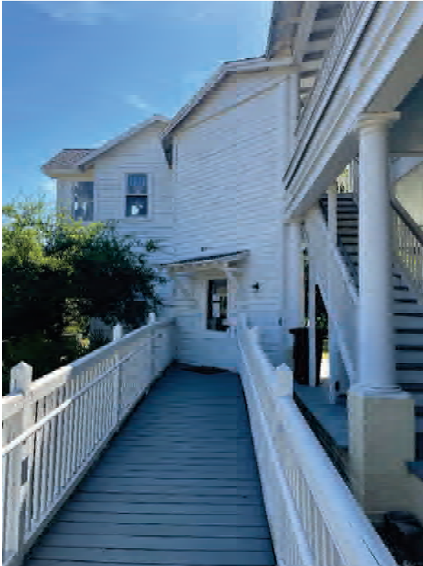
Figure 13, Accessible Ramp: Manor Public Entrance and Restrooms
