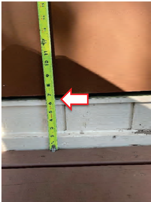
Figures 46 & 47: Classroom Egress Door Clearance and Threshold
