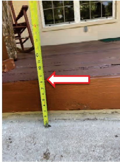
Figure 51, 52, 53: ADA Cottage #3 Step Landing, Risers
