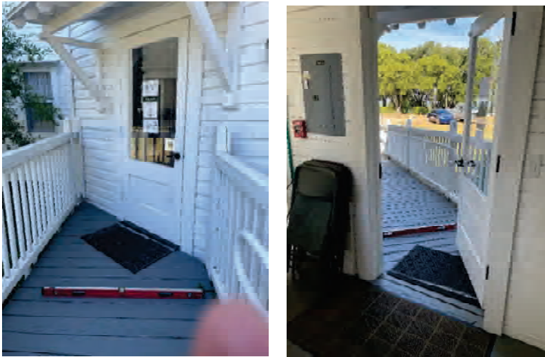
Figure 25, Clear Door Area / Landing
