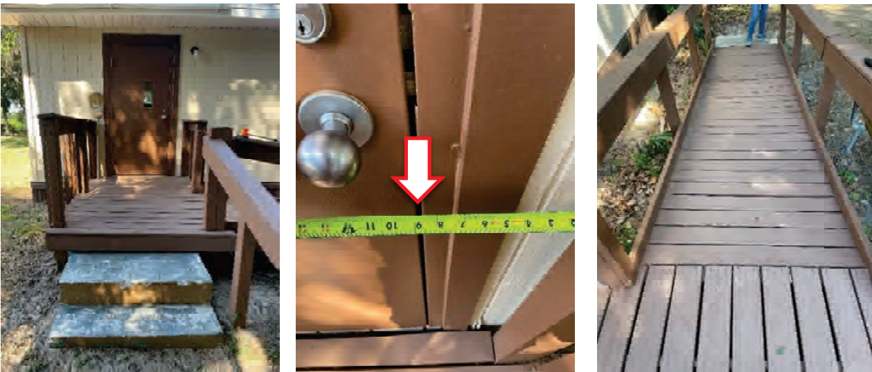
Figures 41, 42, & 43: Classroom Stair, Landing, Clearance and Ramp
