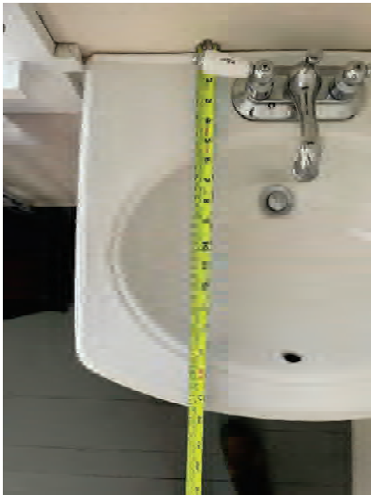
Figures 31 & 32: Lavatory: Depth & Offset from wall
