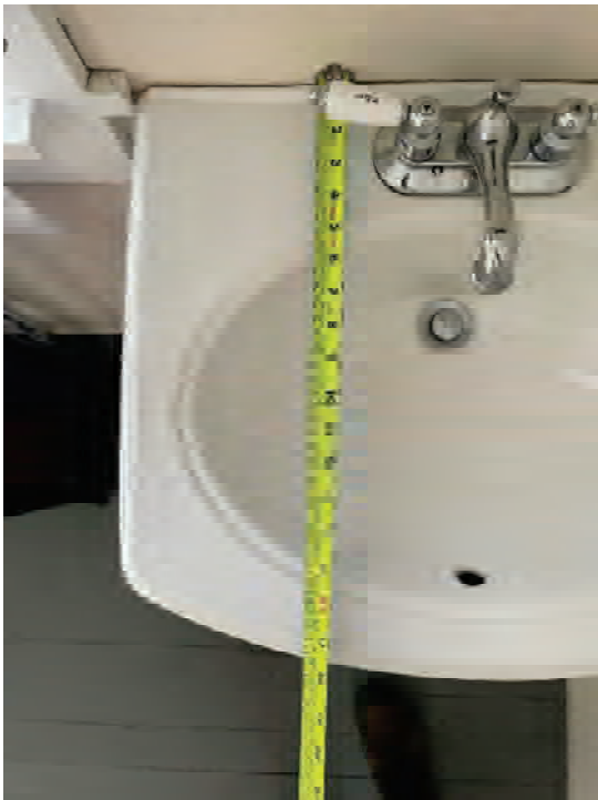
Figures 31 & 32: Lavatory: Depth & Offset from wall
