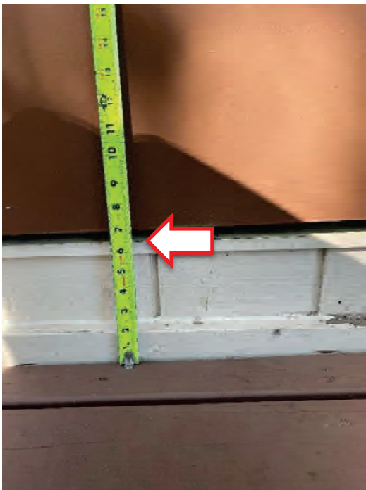
Figures 46 & 47: Classroom Egress Door Clearance and Threshold
