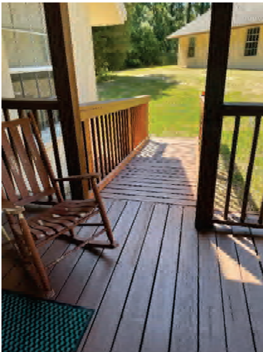
Figure 49: ADA Cottage #3 Location L Ramp
