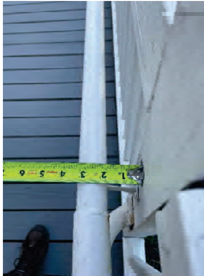
Figure 17, Handrail Clearance and Diameter
