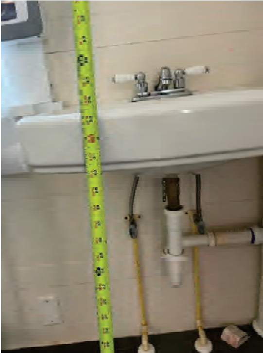
Figures 33 & 34: Lavatory: Height and Scald Protection
