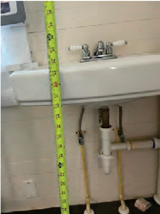
Figures 33 & 34: Lavatory: Height and Scald Protection
