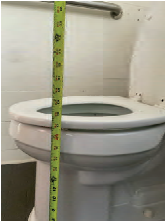
Figures 27 & 28: Water Closet Height, Offset from wall
