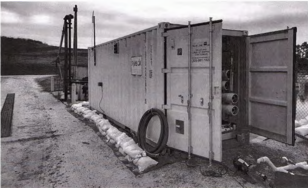
Figure 2-2. ROBOX System Deployed for an Emergency Short-term Treatment Project at a Florida Landfill.
