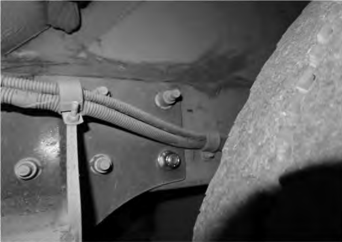
BROKEN HUCK BOLT REPLACED (11,491 TEST MILES)
