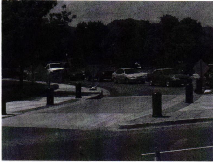
Figure 77 | Raised Crosswalk at Channelized Right Turn
