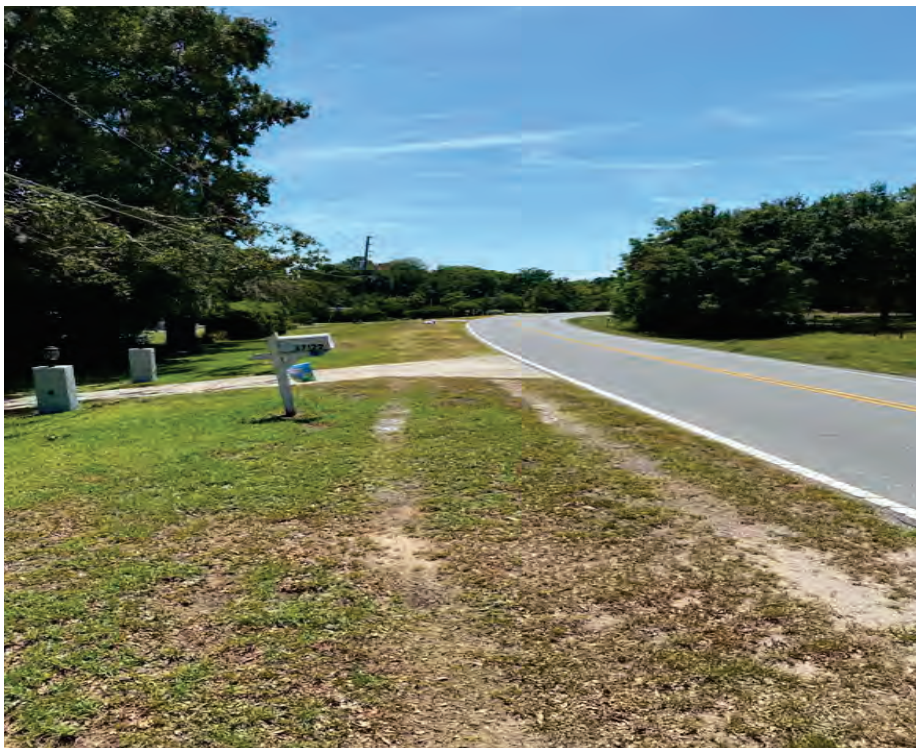
Offtracking on shoulders will be improved through addition of paved shoulders.
