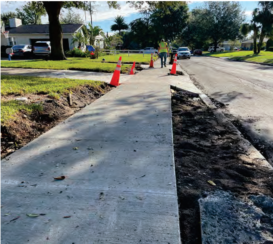
ADA improvements included at driveways along with addition of new sidewalk.
