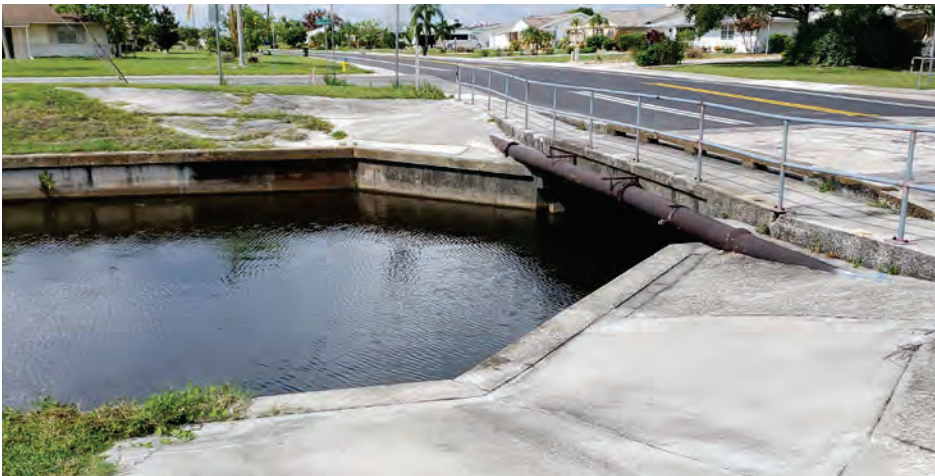
■ Colson Rd Culvert Replacement
