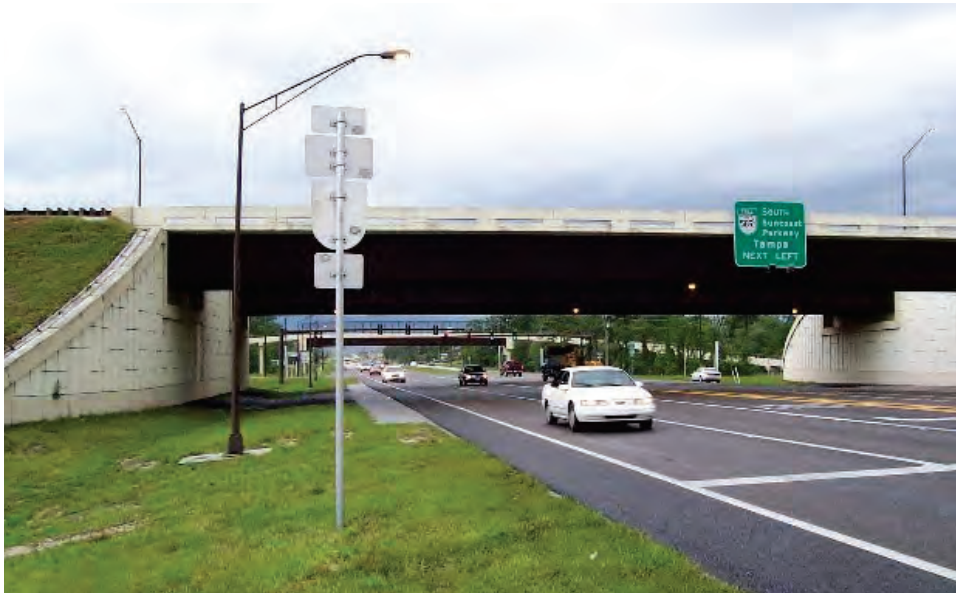
SR 50 (Cortez Boulevard) Widening
