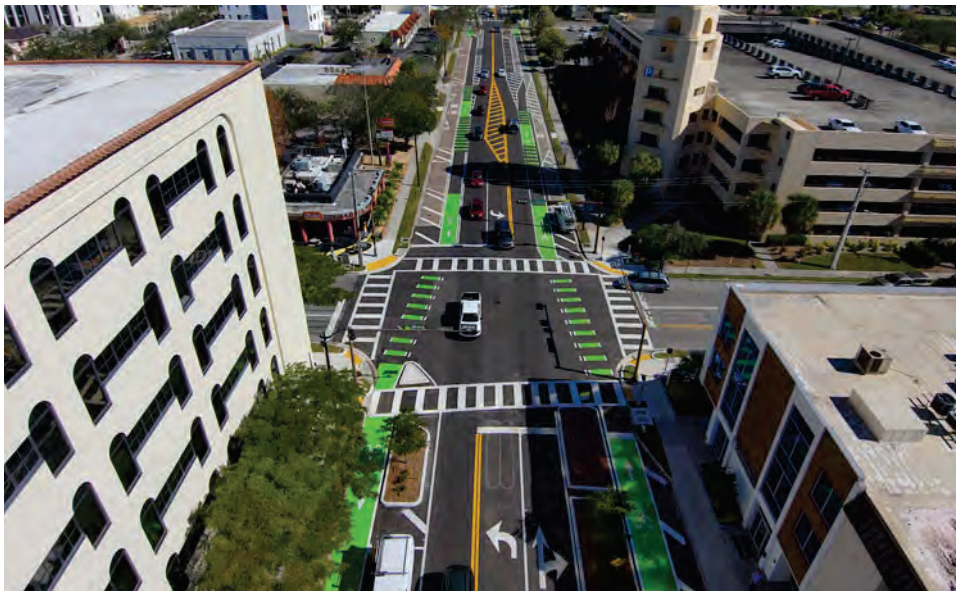
City of Sarasota - Ringling Trail Design-Build Project - East Ave
