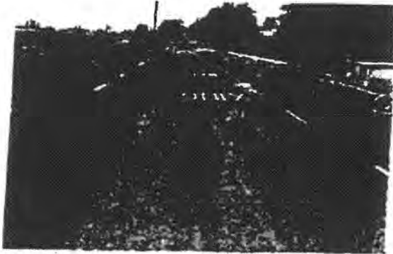
Reclamite was used as a construction seal on the dry areas of this pavement. Untreated areas are still wet from water penetrating the surface.
