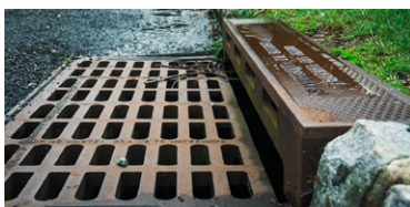
Storm Water Drain
