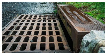
Storm Water Drain
