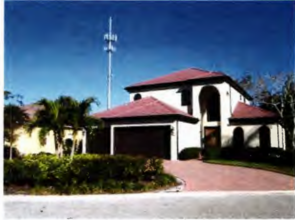
View of tower from cul-de-sac
