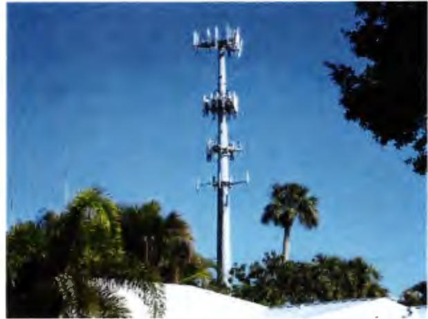
View of tower in front of 304 61 st Street
