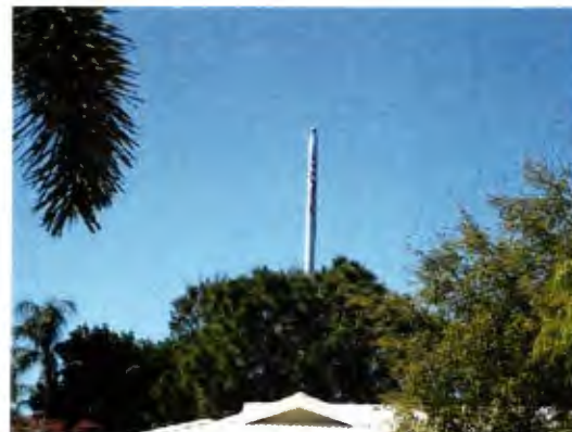
View of tower from front of home
