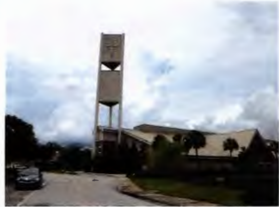
Street view of bell tower installation
