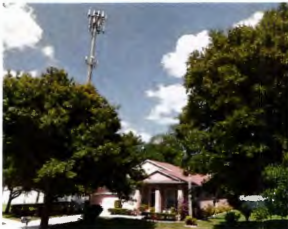
1481 Falconcrest Boulevard and tower 50 feet to the north
