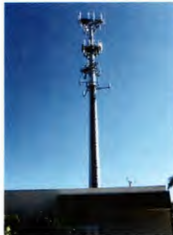
View of tower from the front of 312 and 314 60 th Street
