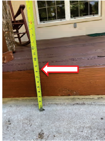
Figure 51, 52, 53: ADA Cottage #3 Step Landing, Risers
