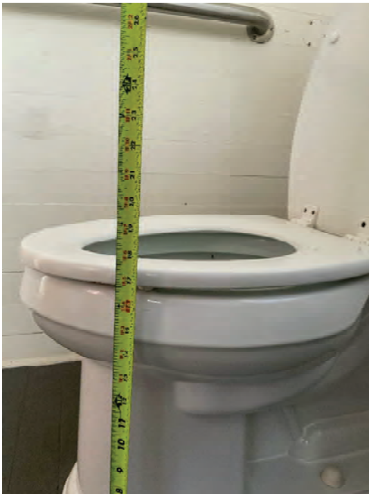
Figures 27 & 28: Water Closet Height, Offset from wall
