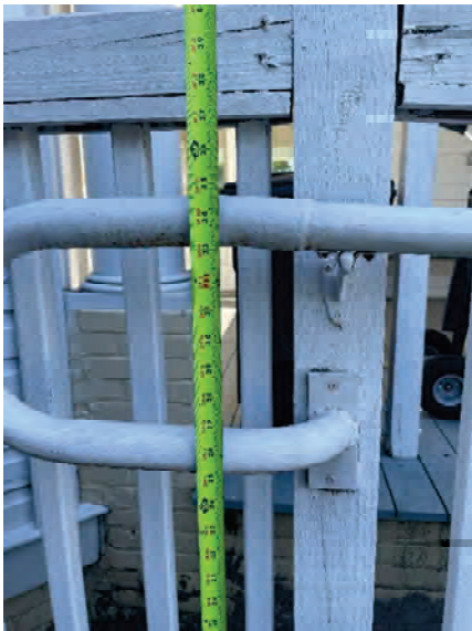
Figure 18, Handrail Extension
