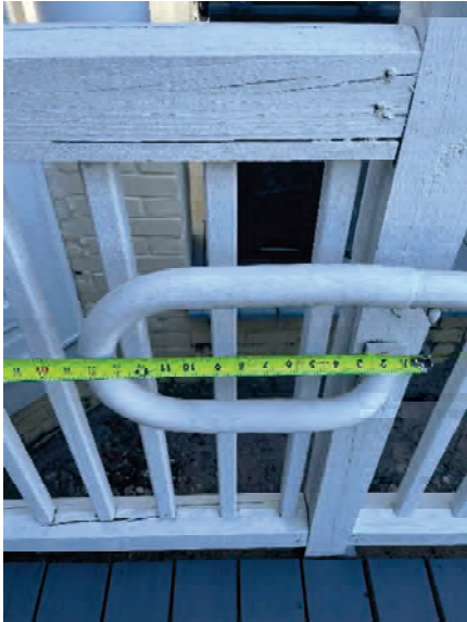
Figure 16, Handrail Return
