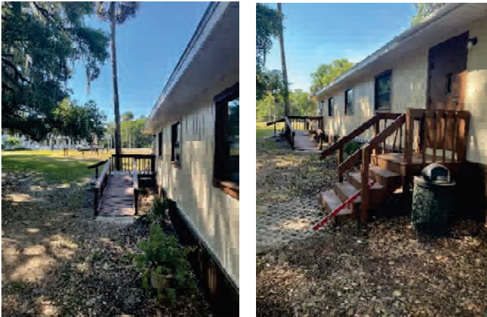
Figures 39 & 40: Path from Manor to Classroom, Egress Ramp and Stairs
