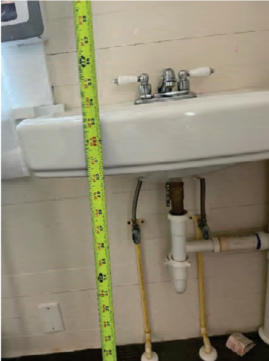
Figures 33 & 34: Lavatory: Height and Scald Protection
