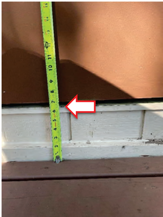
Figures 46 & 47: Classroom Egress Door Clearance and Threshold
