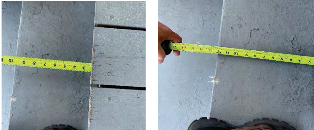
Figure 23 & 24 Step Tread Depth and Nosings
