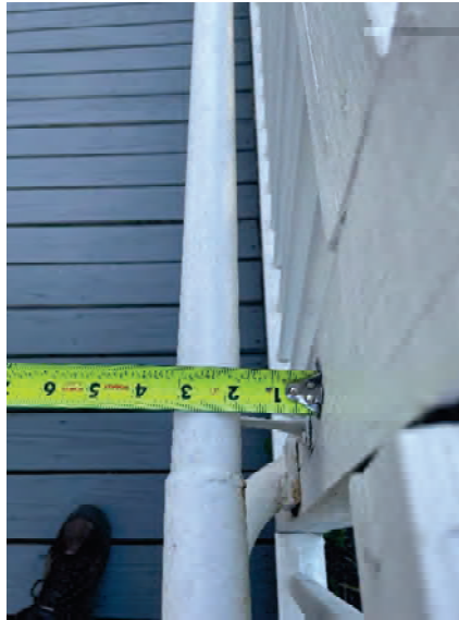
Figure 17, Handrail Clearance and Diameter
