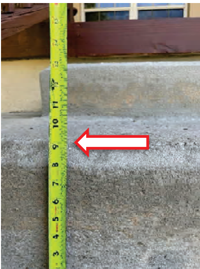
Figure 54, 55, 56: ADA Cottage #3 Step Risers and Treads
