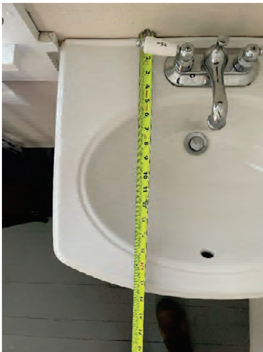
Figures 31 & 32: Lavatory: Depth & Offset from wall
