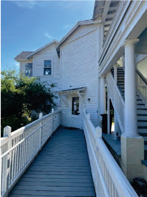
Figure 13, Accessible Ramp: Manor Public Entrance and Restrooms
