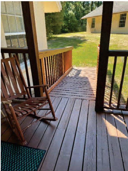
Figure 49: ADA Cottage #3 Location L Ramp
