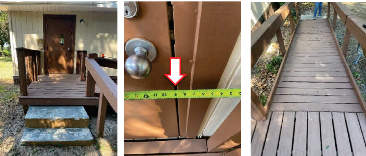
Figures 41, 42, & 43: Classroom Stair, Landing, Clearance and Ramp
