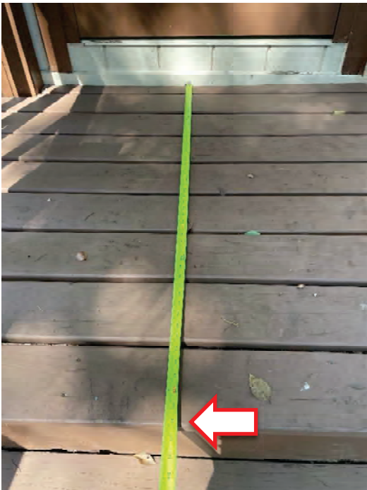
Figures 46 & 47: Classroom Egress Door Clearance and Threshold
