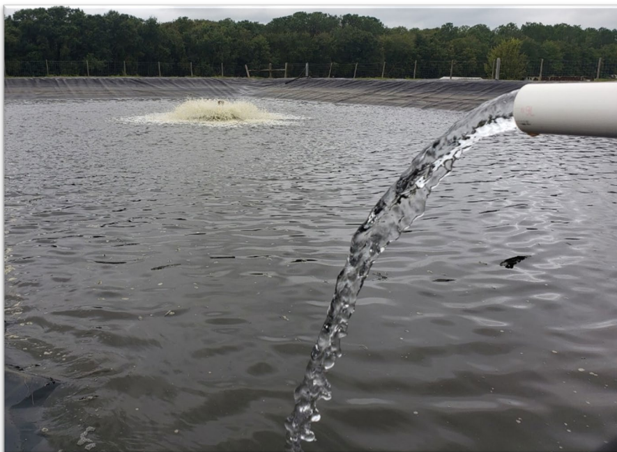
Figure 4-1. Permeate from the Reverse Osmosis Leachate Pre-Treatment System at New River Regional Landfill
