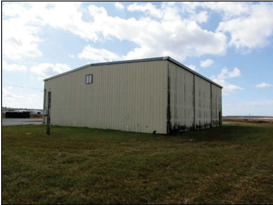
SUBJECT PROPERTY BLDG REAR SEEN FROM THE NORTH
