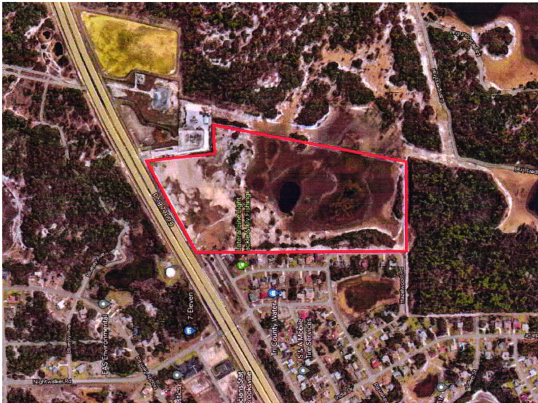
FIGURE 1: Clever Cow LLC - PARCEL KEY #s 1170618 & 346717 - Aerial SUBJECT PROPERTY
