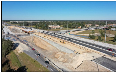
Roadwork on State Road 50; source: Tampa Bay Times.
