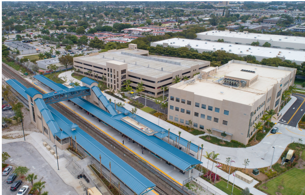
SFRTA Operations Center, Pompano Beach, FL
