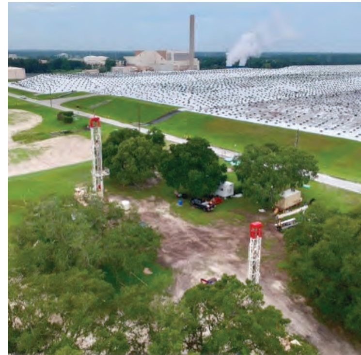
Pasco County Landfill Leachate Wells
