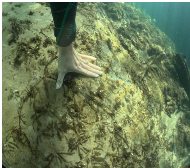
Figure 4. Example of unprotected units showing signs of lateral expansion.
