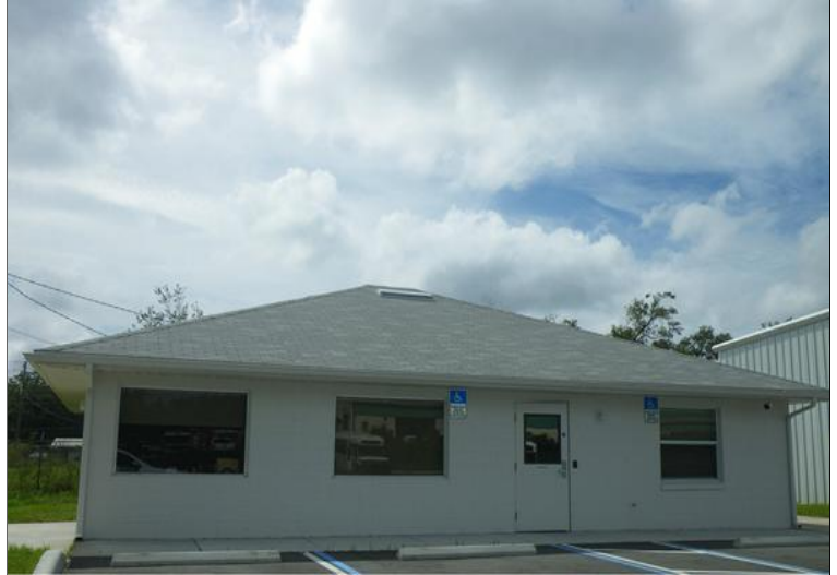
October 2017 BUILDING 01 PHOTO
