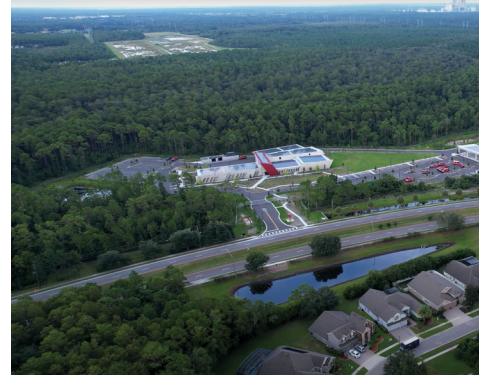
OC Fire Rescue Training Center
