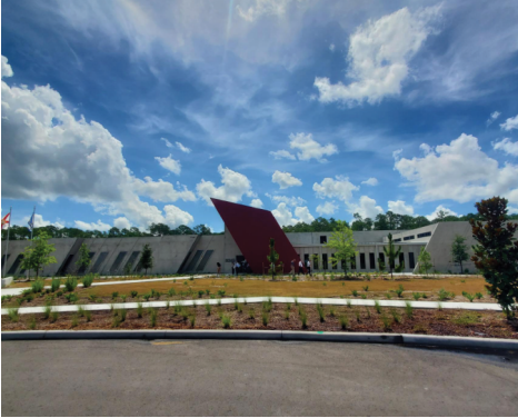
OC Fire Rescue Training Center
