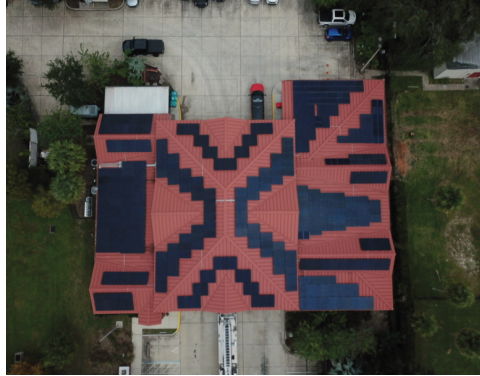
City of Orlando Fire Station 07 Solar Panels
