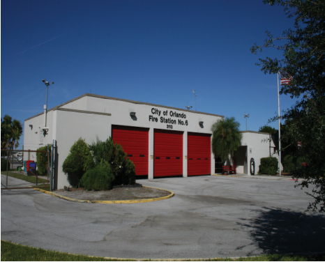
City of Orlando Fire Station 06 Reroof
