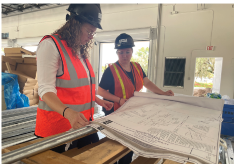
Lex and Sabrina on Site at OC Mosquito Control Facility
