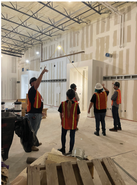
KMF on site at Orange County Mosquito Control Facility
