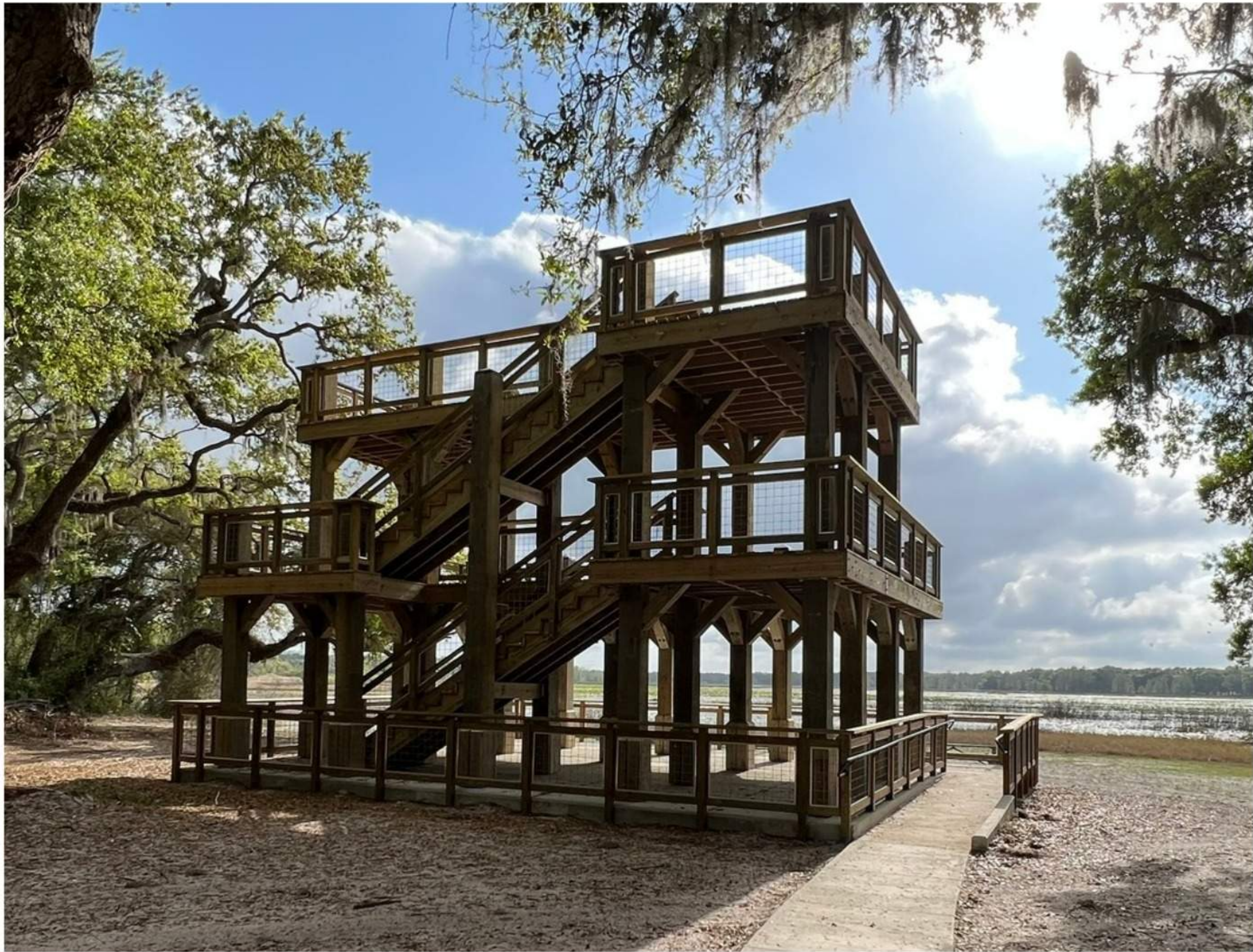
Crews Lake Observation Tower
